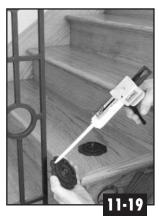
Medallions consist of two halves that screw together. Apply epoxy adhesive on the screw and contact points. **PHOTO 11-19.**
