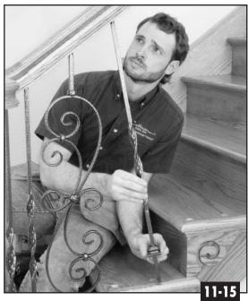
With the base collar placed on the bottom of the baluster, work the baluster into place by inserting the top of the baluster into the rail hole and sliding the bottom of the baluster over and down into the tread hole. **PHOTO 11-15.**
