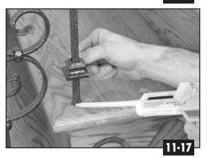
Finish installation by using epoxy to fill any void around the base of the baluster and to secure the base collar. **PHOTO 11-17.**
