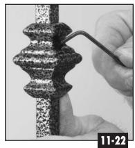
After the balusters are installed, use an allen wrench to tighten the collar's set screw, permanently attaching the collar at the desired location. **PHOTO 11-22.**
